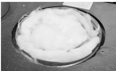
**Step 3:** Remove insulation from inside flue pipe.
