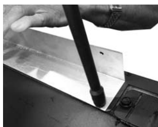
Step 2: Remove the three screws that align with the clearance screw holes from the top of the unit. Secure the center bracket to the top center of the fireplace
