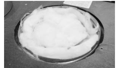
Step 3: Remove insulation from inside flue pipe.
