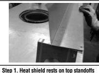
The heat shield is designed to protect framing.
