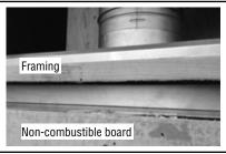
Step 3. Heat shield will now protect framing from heat from flue.
