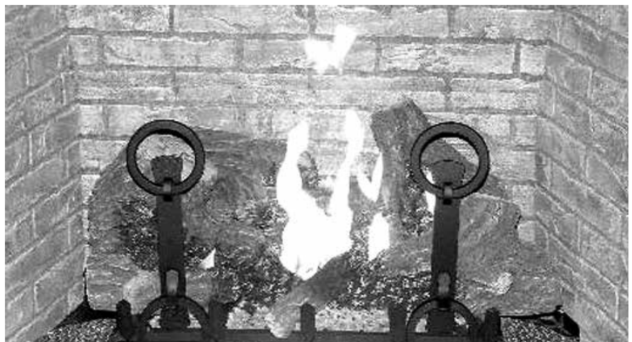
Figure 43 - Burner Flame Appearance
